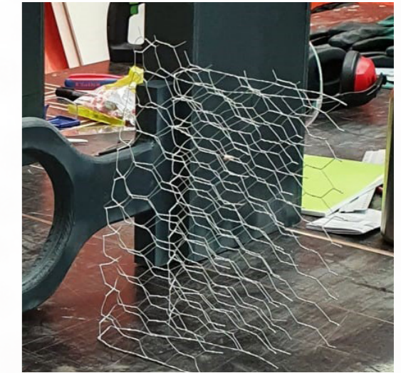
Adding chicken wire inside the storage and spraypainting the system
